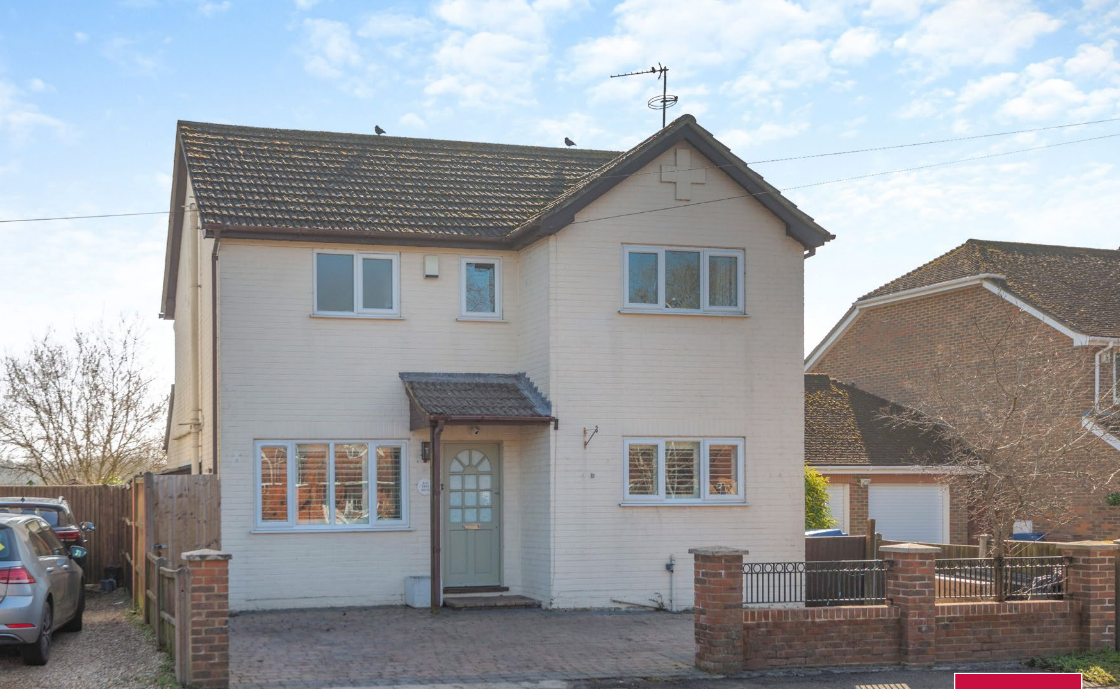
Bay Tree House North Street, Winkfield, Berkshire
