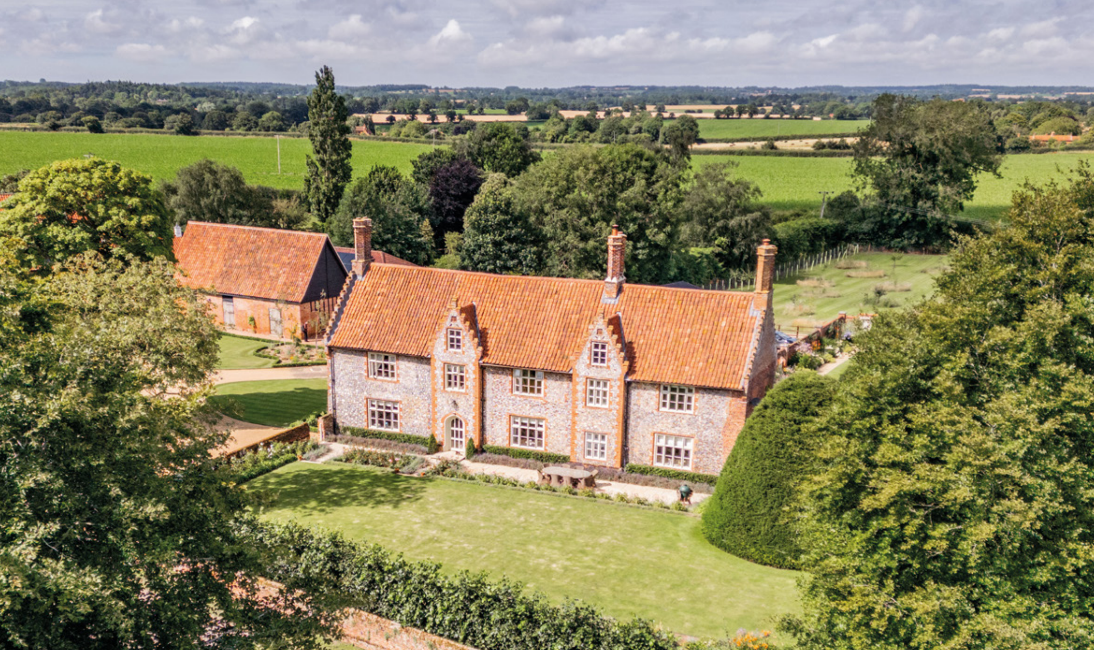
Churchgate House, Wood Dalling, Norfolk
